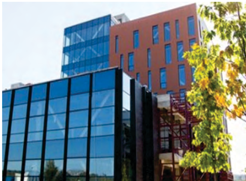
Photo caption: First Tower of Digital Park. Photo credit: MCP
