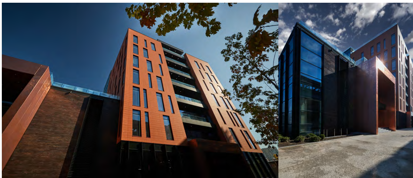
Photo Caption: Moldova IT Park building Photo Credit: Moldova IT Park
